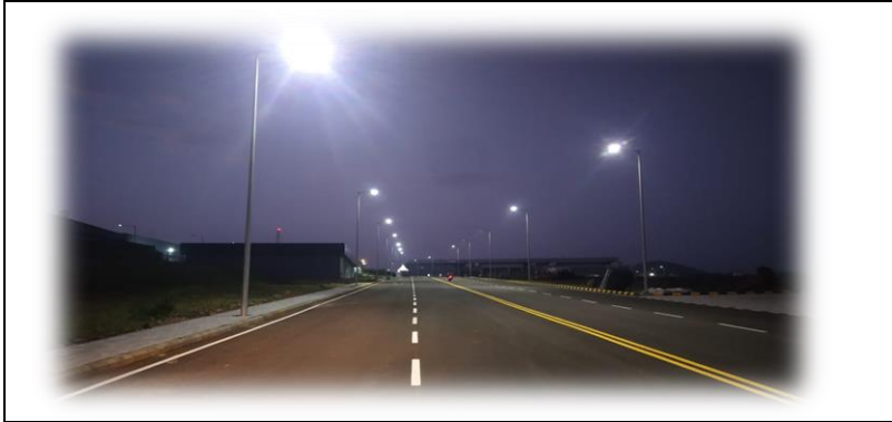
External Lighting - Indospace - Chakan - Pune
